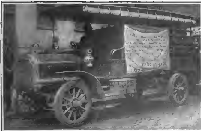
MACK GASOLINE TRUCK WITH MOTOR UNDER HOOD.
